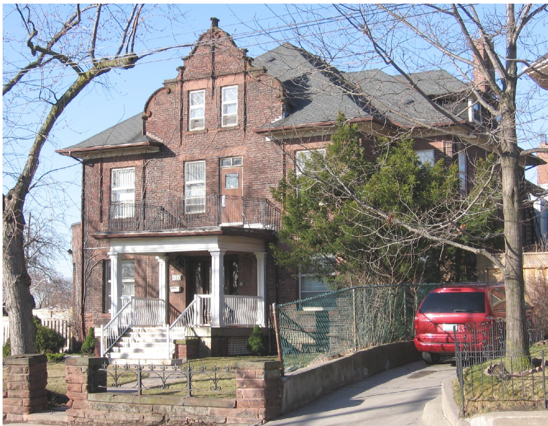
View of the principal (east) façade (left) and north elevation (right), March 2010
