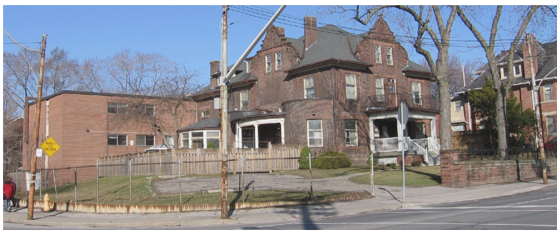
View of the principal (east) façade facing Pape Avenue (right) and the south elevation overlooking Riverdale Avenue (left)
