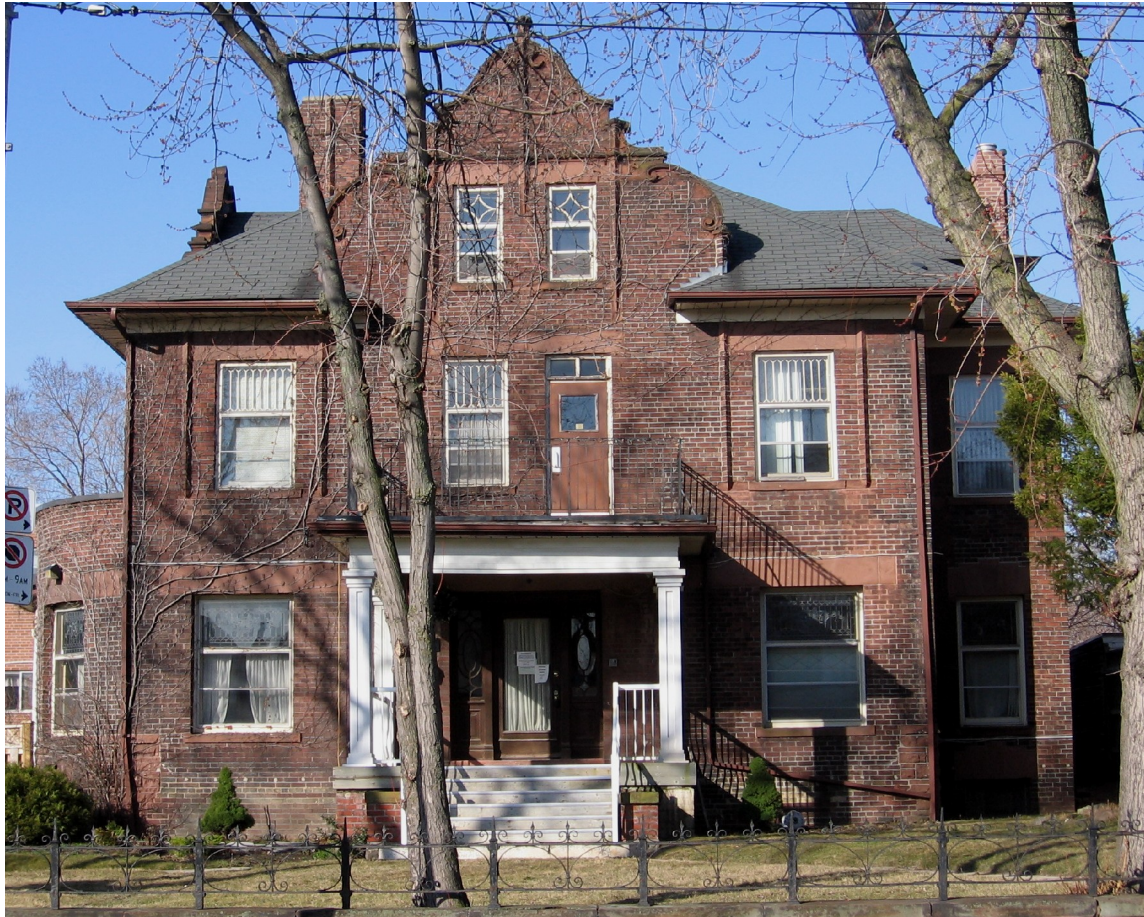
Principal (east) façade
